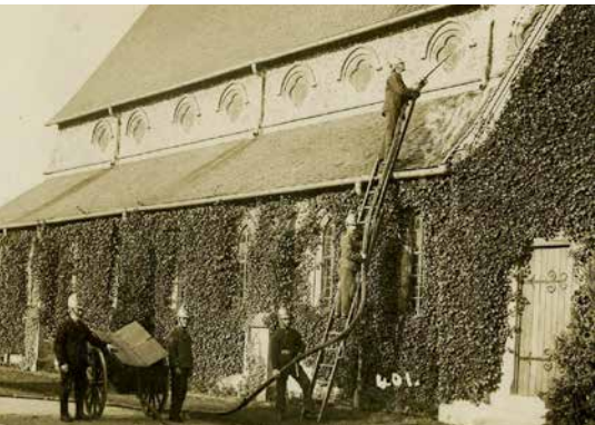
Fire practice at the war hospital. Two of the men are orderlies, with a Red Cross on their right sleeve. Graylingwell had its own fire-fighting equipment. Image courtesy of West Sussex Record Office, Acc 18161
